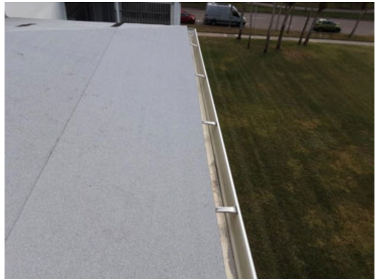
Lower Roof 2 - Gutters
