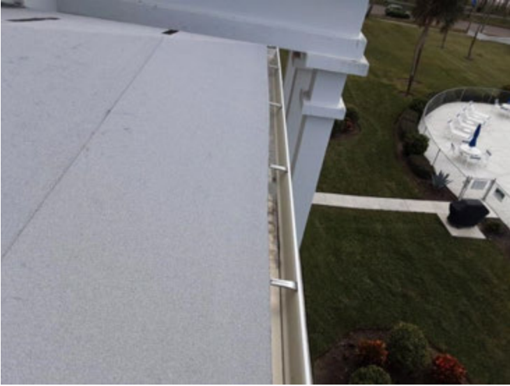
Lower Roof 4 - Gutters
