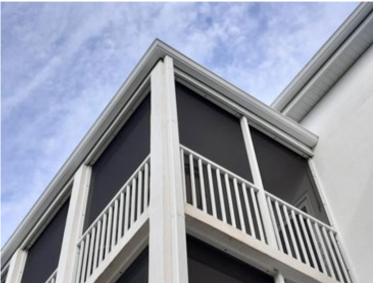
Lower Roof 3 - Downspouts
