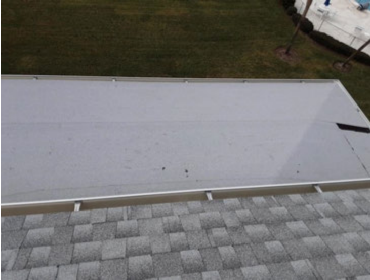
Lower Roof 3 - Appearance Overview The appearance of the roof is in good condition.
