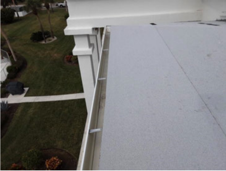
Lower Roof 2 - Gutters
