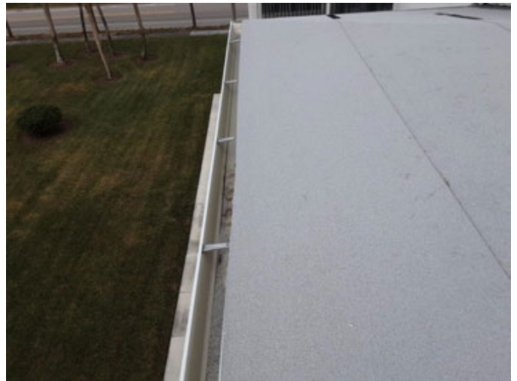
Lower Roof 4 - Gutters
