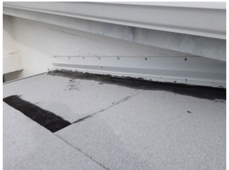
Lower Roof 2 - Membrane Overview The membrane appears to be in good condition.
