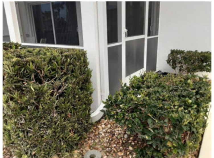
Lower Roof 1 - Downspouts
