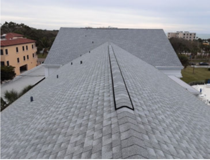
Roof Overview General roof overview
