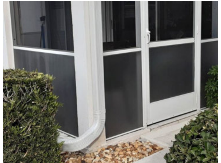
Lower Roof 3 - Downspouts
