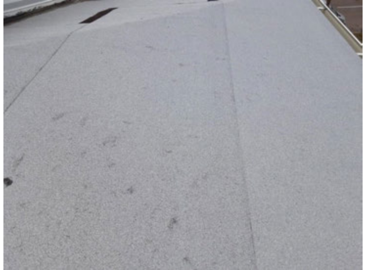
Lower Roof 3 - Membrane Overview The membrane appears to be in good condition.
