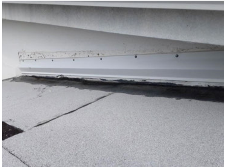
Lower Roof 3 - Membrane Overview The membrane appears to be in good condition.
