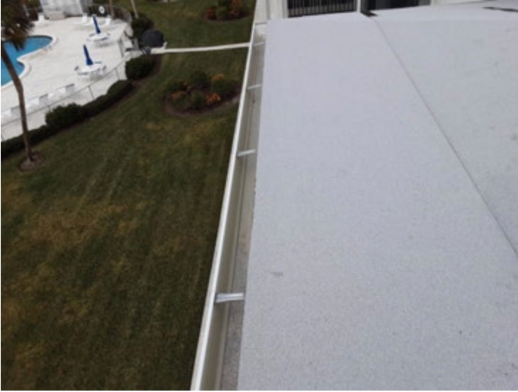
Lower Roof 3 - Gutters
