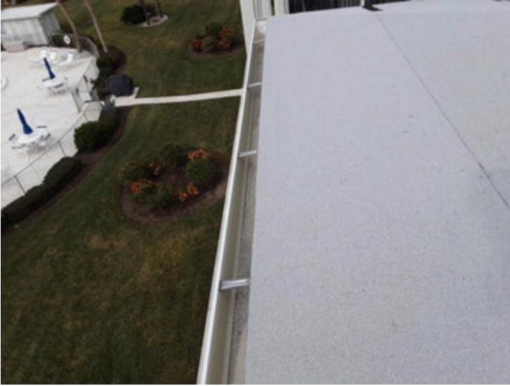
Lower Roof 1 - Gutters
