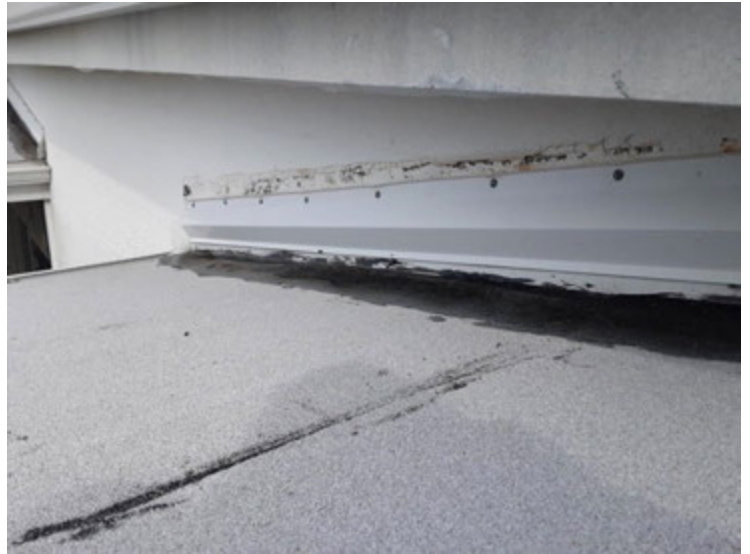
Lower Roof 1 - Membrane Overview The membrane appears to be in good condition.
