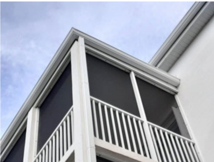
Lower Roof 2 - Downspouts
