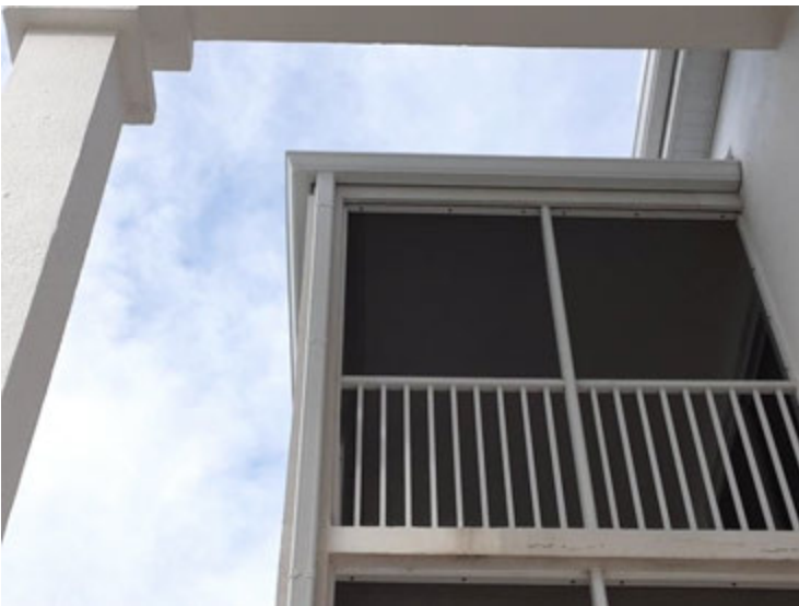
Lower Roof 4 - Downspouts
