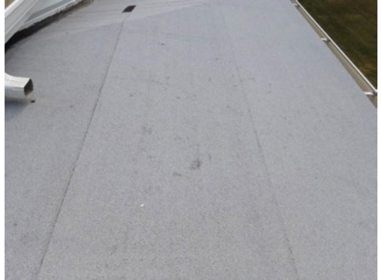
Lower Roof 2 - Membrane Overview The membrane appears to be in good condition.
