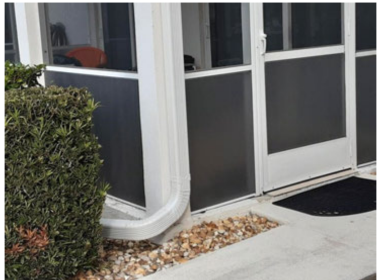
Lower Roof 2 - Downspouts
