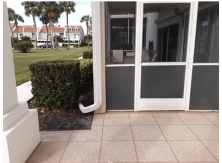
Lower Roof 4 - Downspouts
