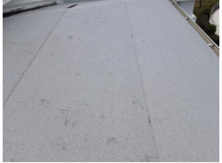
Lower Roof 4 - Membrane Overview The membrane appears to be in good condition.
