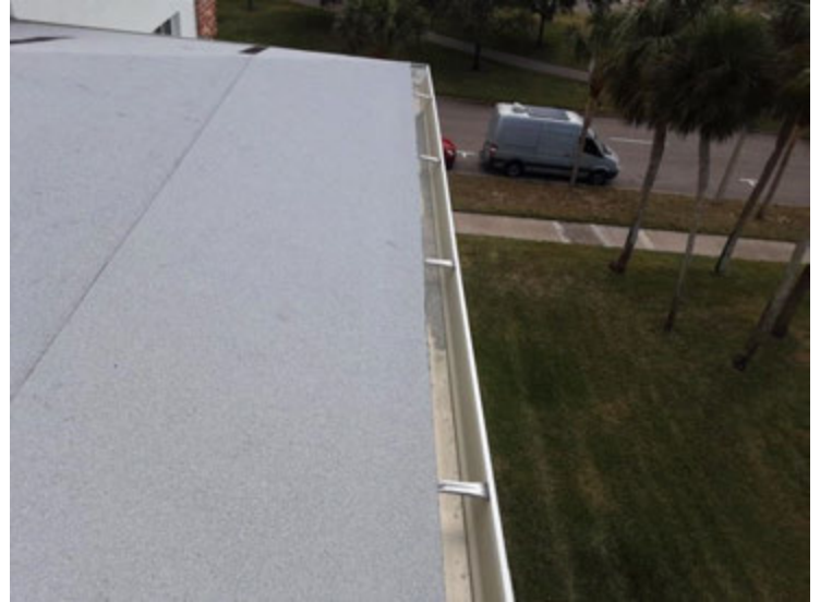
Lower Roof 3 - Gutters
