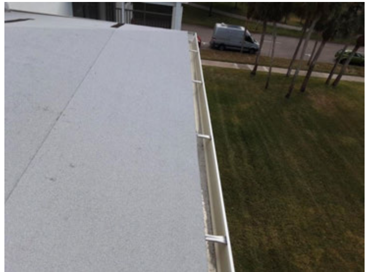
Lower Roof 1 - Gutters
